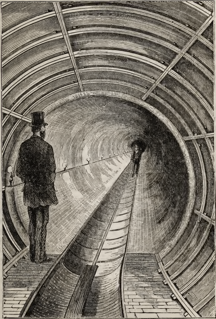
TUNNEL UNDER BROADWAY.
